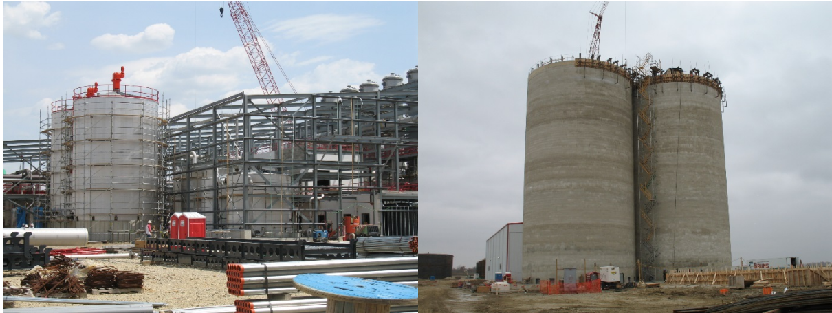
Cardinal Ethanol under construction 2007-2018:
